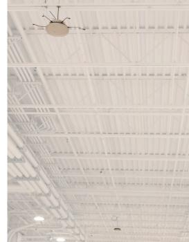
Nine Adiatec FA-3 fan-assist units above the plant floor disperse atomized water for humidification and evaporative cooling.
