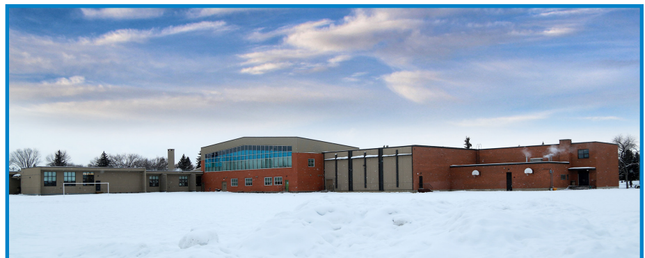
The makeup air unit for the Aurora School gym uses outside air all winter long, furthering the need for humidification.
