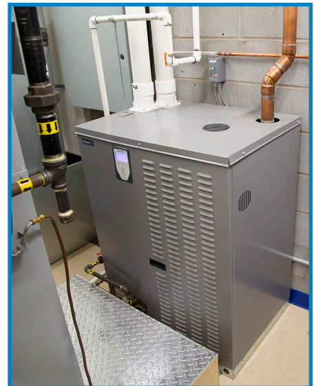
The DriSteed GTS® humidifier LX series was chosen for its small footprint, efficiency, and the low installation cost of PVC venting.
