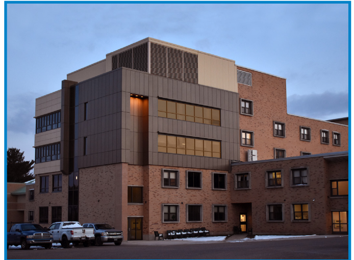
Canal View—Houghton County got a new addition and air handler in 2017.
