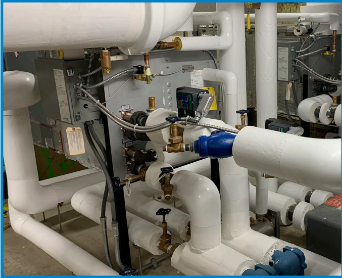
The STS steam-to-steam humidifier uses pressurized boiler steam in a heat exchanger to boil chemical-free water into clean humidification steam.
