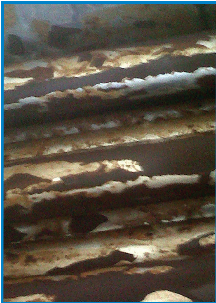
GTS humidifier heat exchanger before de-scaling treatment
