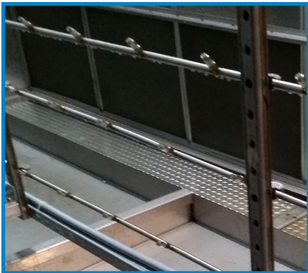
Atomizing nozzles upstream from mist eliminators
