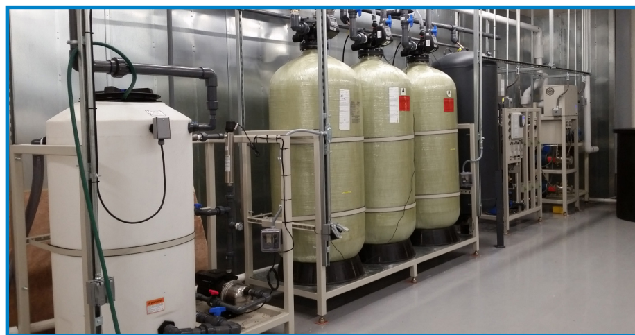
Reclaim tank (far left) for water that does not evaporate in the air handlers
