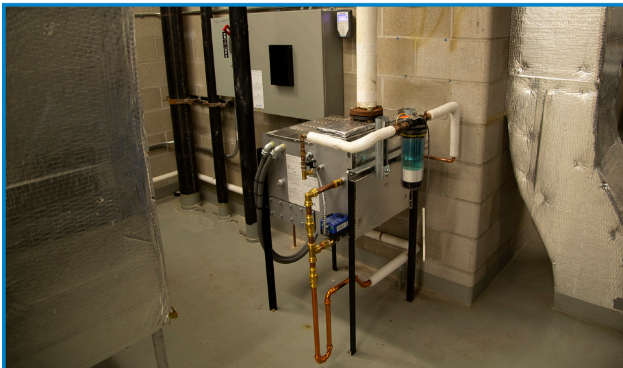
Two Vaporstream® electric steam humidifiers generate a combined 210 pounds per hour of steam, enough to humidify the whole building to a healthy 40% RH.
