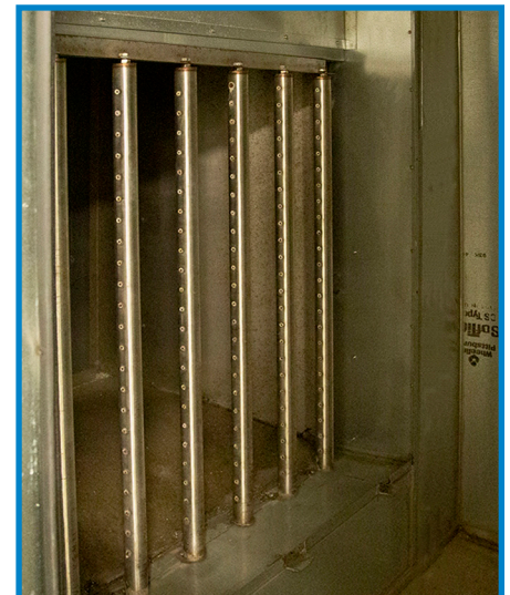
Each of the two air handlers has a Rapid-sorb® steam dispersion panel with 220 steam outlets.
