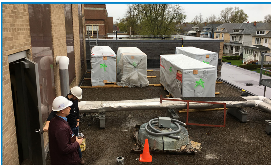
This door is one of the mechanical room egress/access points and the one used for components and site-built options, including DriSteem's 104- by 98-inch Ultra-sorb® LV steam dispersion panels.
