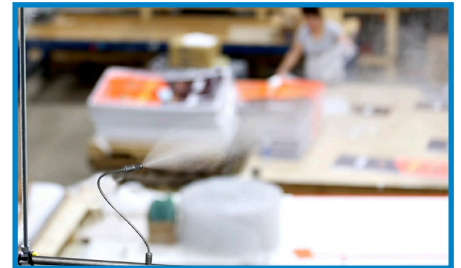
One of the 165 atomizing nozzles in over a quarter mile of tubing throughout Modernistic's 160,000-square-foot facility.
