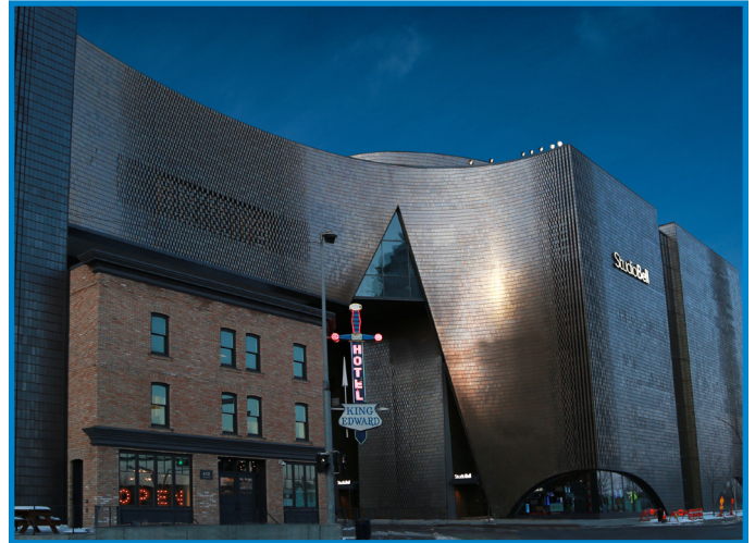
At five stories and 160,000 square feet, Studio Bell dwarfs the 100-year-old King Edward Hotel. The "King Eddy" was scheduled for demolition in 2004, but it was saved in a brick-by-brick restoration and is now a feature of the NMC.
