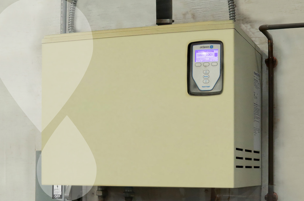
Vapormist electric steam humidifier boils RO water into steam whenever the digital press is running
