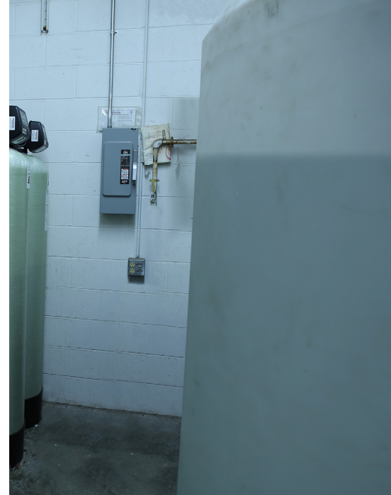
300-gallon RO storage tank supplies humidifier with fill water and press rooms with water for aqueous coatings
