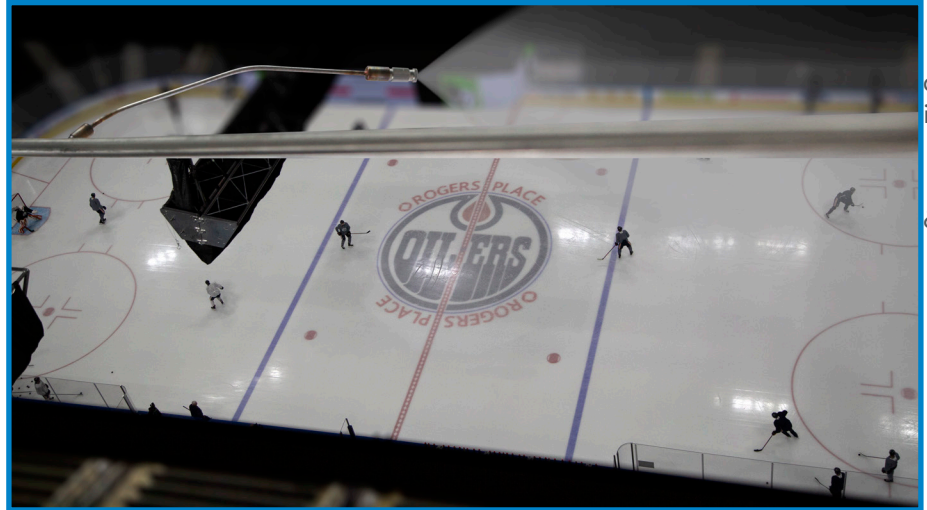
One of 70 atomizing nozzles at the catwalk level of the Rogers Place
