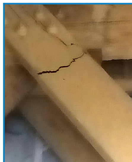
Several dry rotted and cracked trusses were repaired in early 2021.
