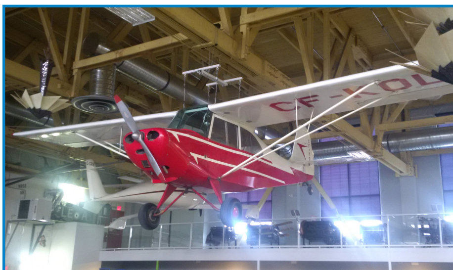
Wooden trusses support the roof and several suspended aircraft displays.
