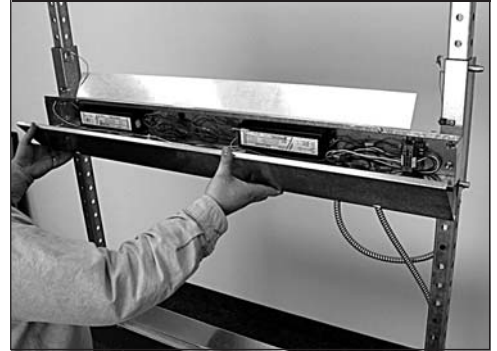
Figure 11-1: Removing fixture cover
