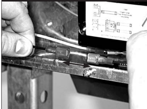
Figure 16-1: Disconnecting quick connects from ballast leads
