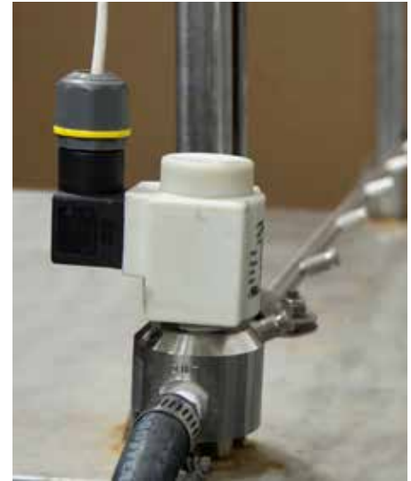
FIGURE 34-1: DRAIN VALVE AND DRAIN PIPING AT END OF MANIFOLD SECTION
