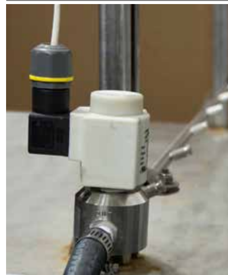
FIGURE 53-1: DRAIN VALVE AND DRAIN PIPING AT END OF MANIFOLD SECTION
