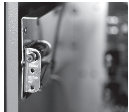
Door interlock switch in control cabinet
