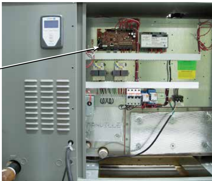
FIGURE 4-2: CONTROL BOARD MOUNTED ON GTS SUBPANEL
