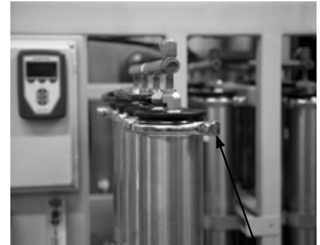
FIGURE 47-1: DRISTEEM REVERSE OSMOSIS MEMBRANES
